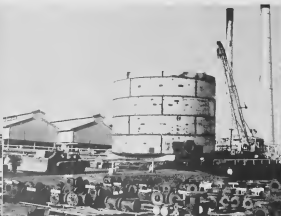
A GIANT mobile crane loovers over the line of march. Shippage on inclines is prevented by the use of two cranes. UN GIGANTESCO grua móvil ta swavi over di ruta. Slipmento na bhadada ta worde prevent usando dos grua.
